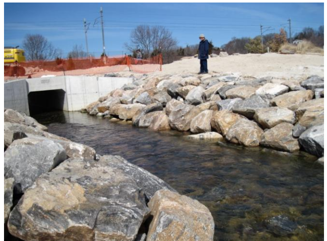
At Rocky Neck, alewives used to have to struggle thru two small pipes to get into Bride Brook. With this new project, they now can use an open channel except for a short culvert that allows beach goers to get across the brook. Construction Supervisor Deb Corcoran of the DEP/Engineering looks on. Fishway. The wooden gate to close the fishway is resting on top of the fishway. One can see the stone façade added to cover the concrete walls.
