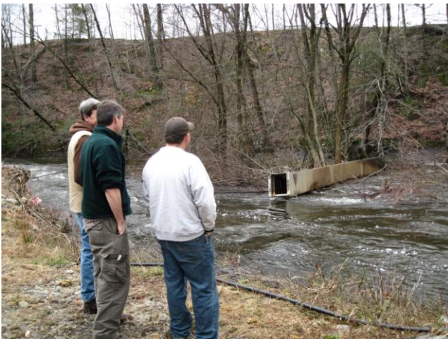
The crew has a "holy crap" moment while looking at the lower section of the Trading Cove Brook fishway, washed 200 feet downstream of the dam in Montville. The lower three sections of steeppasses broke off and will need to be replaced. Left to right: Bruce Williams, Tim Wildman, Dave Ellis.
